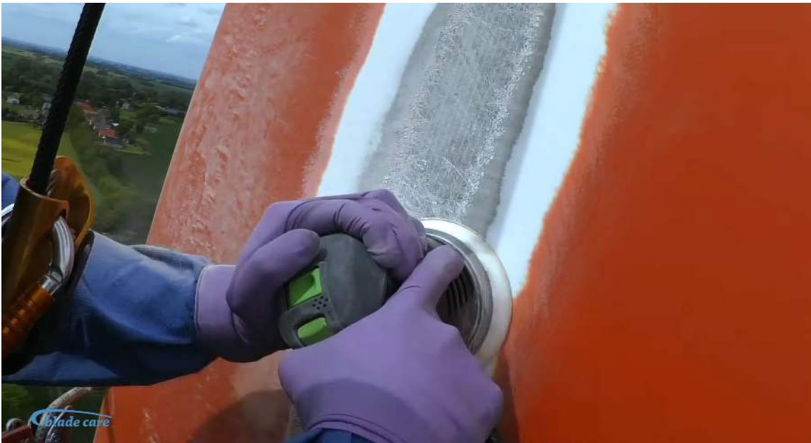
No microplastics pollution here..? Image show the commonly used practice of open air mechanical sanding at an in situ repair job. The industry won't tell you this, but this is common practice. Image from: YouTube.
