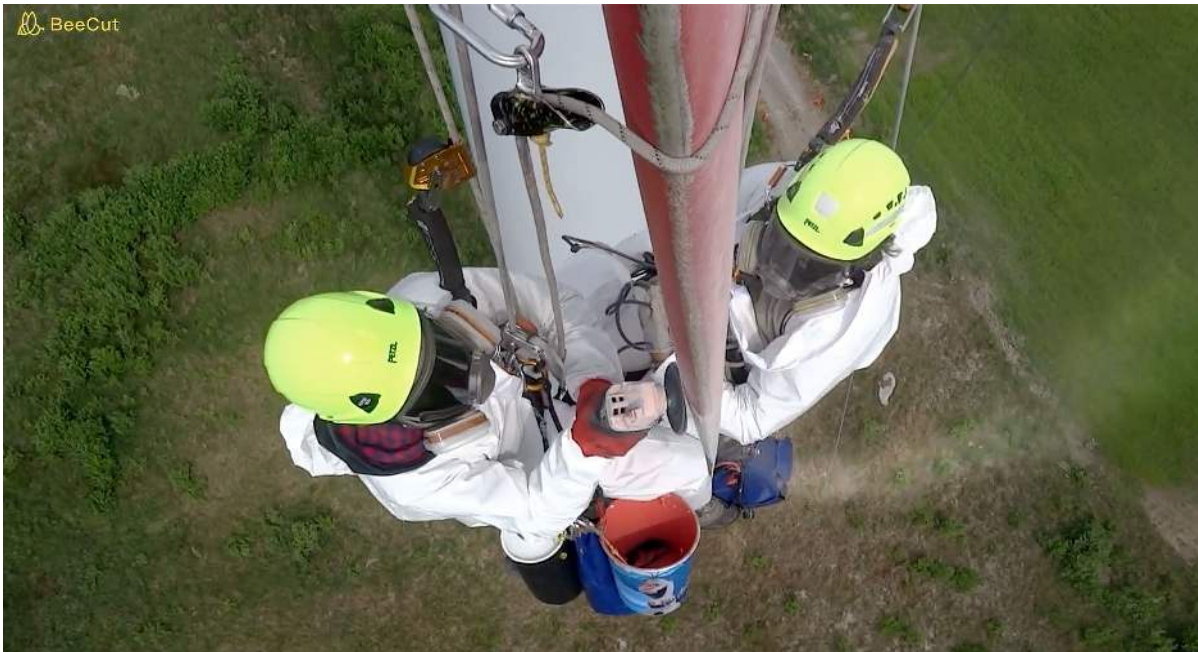
No microplastics pollution here..? Image show the commonly used practice of open air mechanical sanding at an in situ repair job. The industry won't tell you this, but this is common practice. Image from: YouTube.
