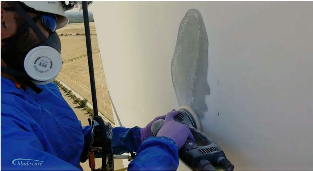
No microplastics pollution here..? Image show the commonly used practice of open air mechanical sanding at an in situ repair job. The industry won't tell you this, but this is common practice. Image from: YouTube.
