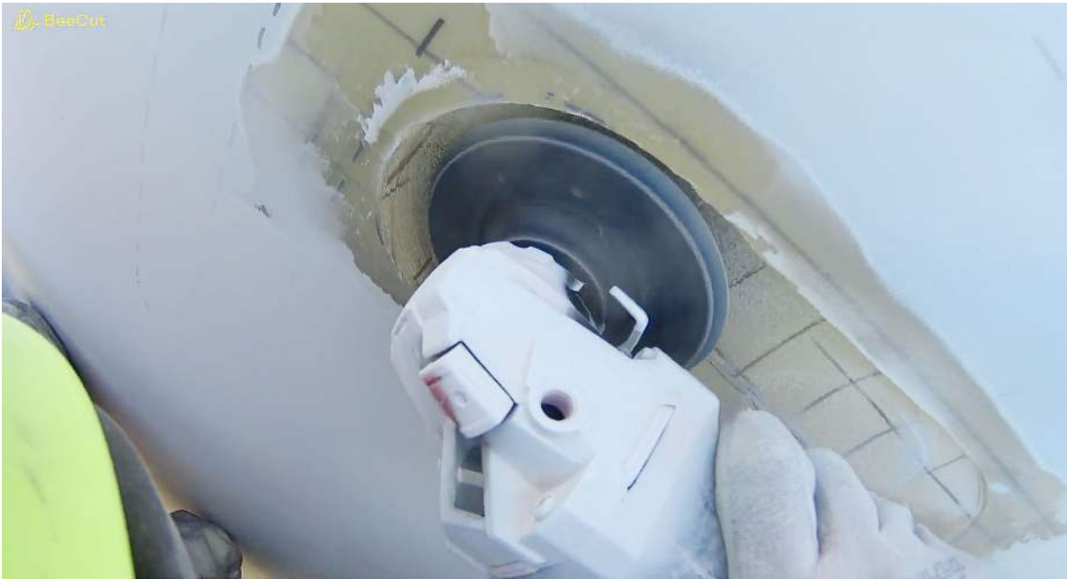
No microplastics pollution here..? Image show the commonly used practice of open air mechanical sanding at an in situ repair job. The industry won't tell you this, but this is common practice. Image from: YouTube.
